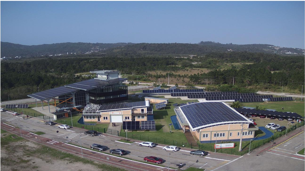
Figure 2 – The Fotovoltaica/UFSC solar energy research laboratory, with the green H<sub>2</sub> laboratory building, which collects rainwater, produces solar electricity and houses the electrolysis system shown in the left-hand corner.
